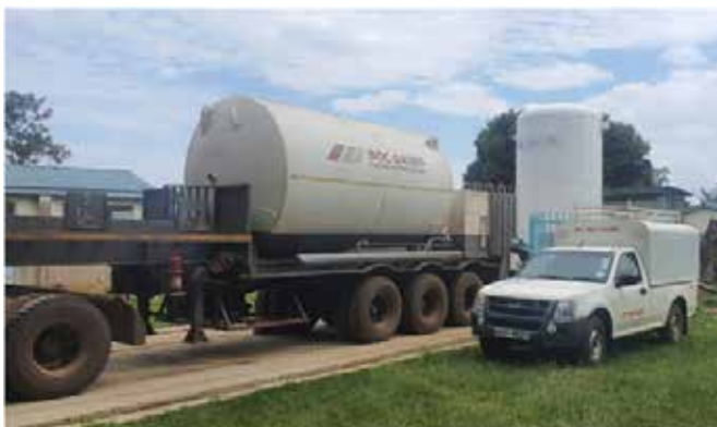
The Tank at Alupe Subcounty Hospital.
