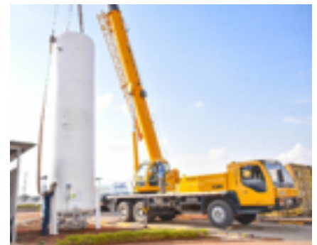
(a) Liquid Oxygen tank (20,000 Litres)- Installation
